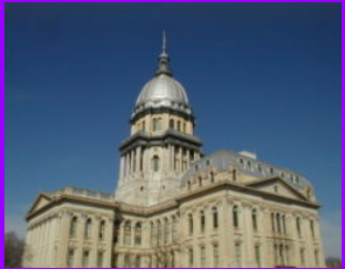
State Capitol Building
